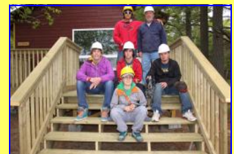
Lasalle students build railings on cabin porches
