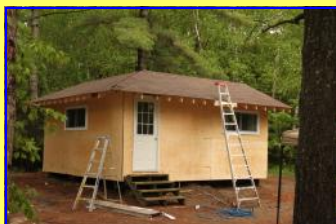
Amatol volunteers completely rebuild Tern cabin
